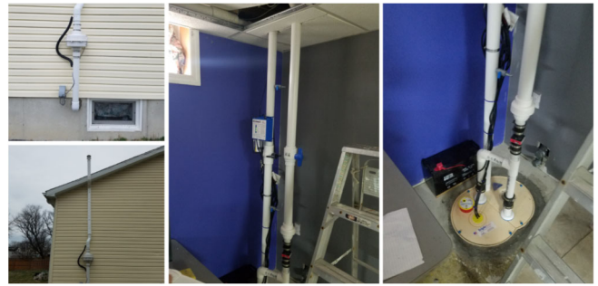
Sub-Slab Depressurization System (SSDS) for vapor mitigation in Vineland, NJ.
